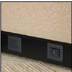
Standard raceways contain built in wireways for data. Allowing data faceplates to be mounted in line with receptacles.
