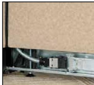
Top feed conduits travel vertically within panels from the ceiling power supply to the raceway where they connect to the panel distribution system.
