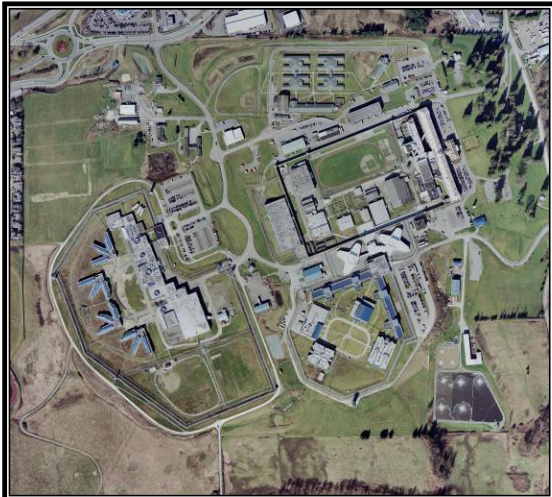
MCC Aerial View
