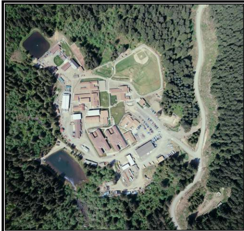
LCC Aerial View
