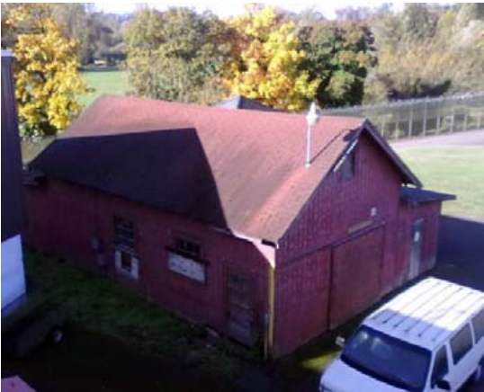
view from above, showing N & E sides 2011
