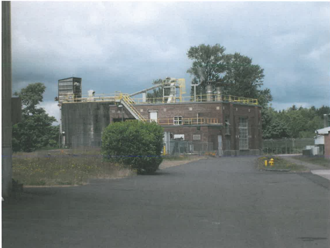
Photograph 3: Central steam plant on southern portion of subject property.
