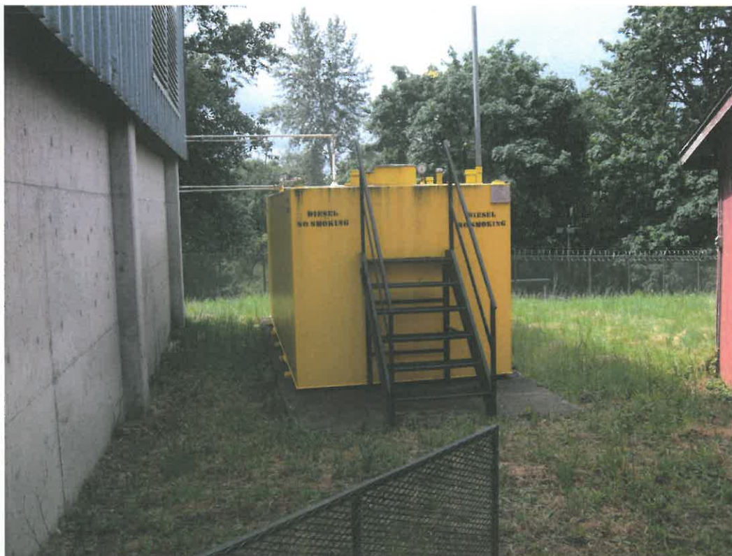
Photograph 4: Diesel fuel AST on west side of steam plant building.
