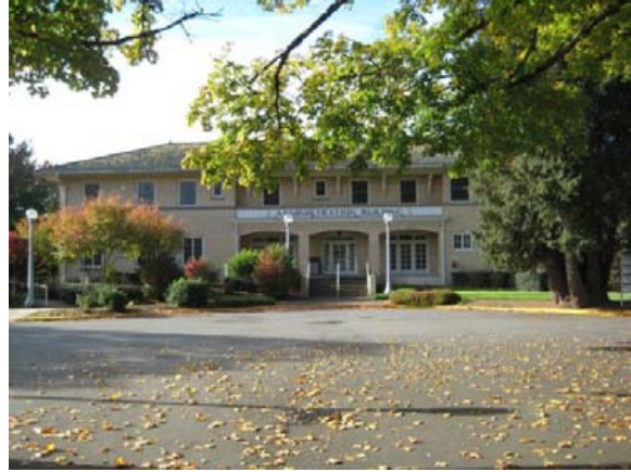
note original lamps around end of entry lane primary N facade 2011
