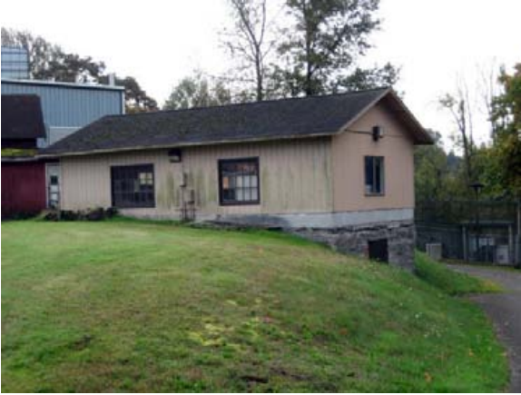
note how building is set into small hill looking SE, showing N & W sides 2011
