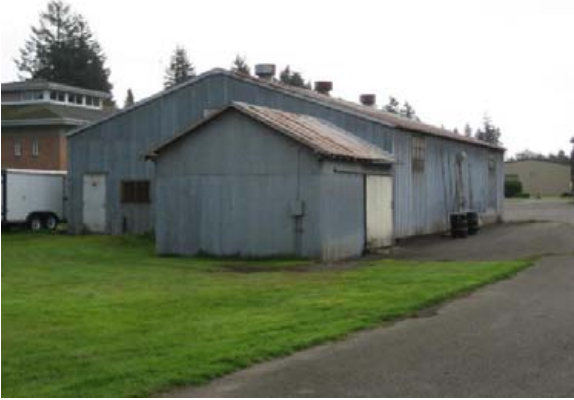
looking E, showing W side and oblique view of S side 2011
