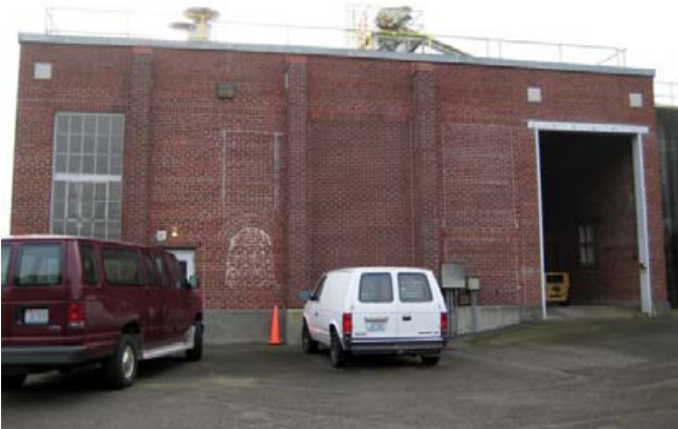
note drive-through south bay, infilled openings W facade 2011
