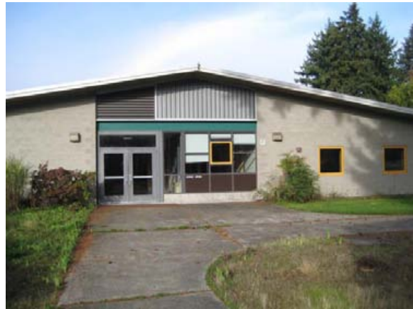
E facade, school portion 2011
