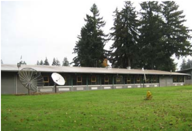
S facade of school portion 2011
