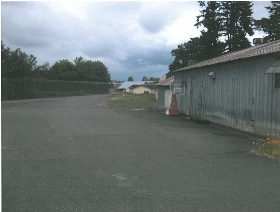
Photograph 6: Asphalt patching indicates former fleet fueling USTs location.
