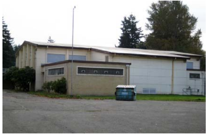
W & partial view of N facade, gym portion 2011
