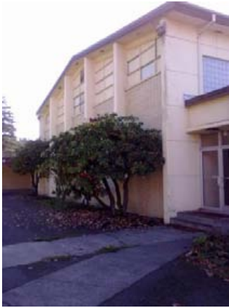
N facade, gym portion 2011
